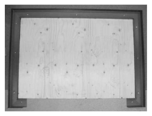
Once you are satisfied with the level the U channel can be rawl-plugged or hilti-nailed into position ensuring it is sealed with silicone sealer between the floor and the channel to prevent moisture penetration. Apply 'mastic sealer' to the inside of the channel so that when the panels are located there is a vapour seal.
