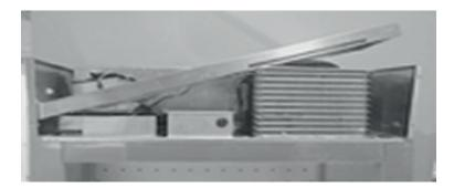
With the ceiling panel in place slide the galvanised angle bracket into place (see fig 4). Secure using the screws provided (see fig 5 and 6).
