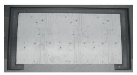
Once you are satisfied with the level, the U channel can be rawl-plugged or hilti-nailed into position, ensuring it is sealed with silicone sealer between the floor and the channel to prevent moisture penetration. Apply 'mastic sealer' to the inside of the channel to provide a vapour seal when the panels are located.
