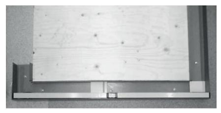
It is recommended that there should be no more than 3mm tolerance in the floor level, as this can affect the correct location of the panels.
