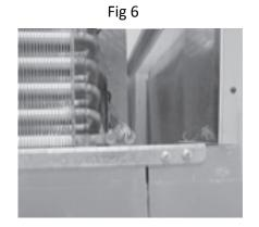
With the ceiling panel secured in place seal the internal joints with silicone sealer. Insert the buttons into the lock holes.
